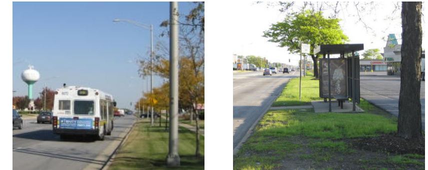
Pace bus service in the Corridor is primarily provided by Route 386, which travels along Harlem and Oak Park Avenues through the Corridor communities. Pace has recently explored upgrading the service and customer facilities along the route as part of its Arterial Rapid Transit initiative (see sidebar, page 3-6).
